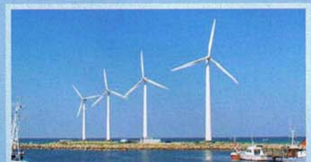
Wind-diesel system at Bønnerup Harbour, Denmark
